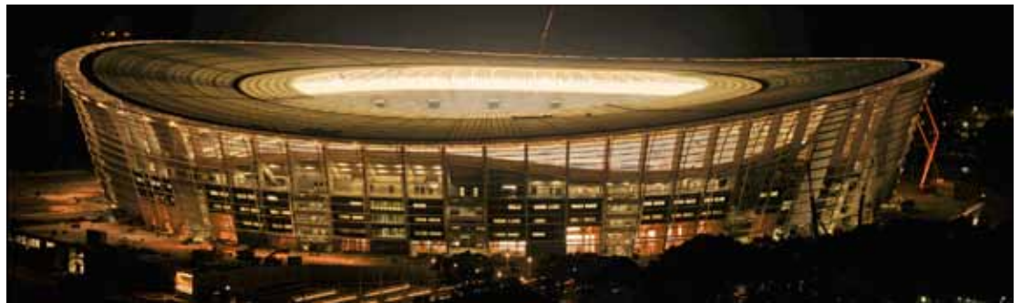
"Cape Town stadium" - DSE fabricated the roof steelwork excluding the compression ring for the new Cape Town stadium, built for this year's FIFA World Cup.
